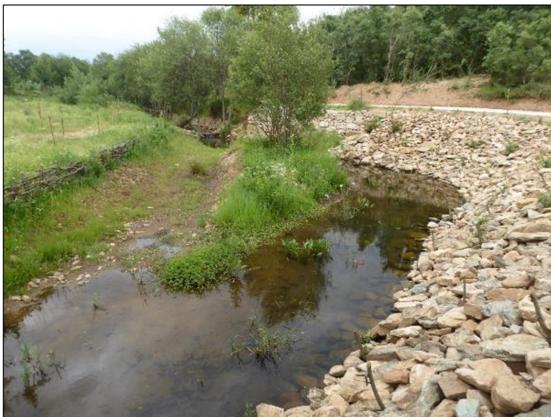
Figure 11-4 Natural bank stabilisation techniques created under Amarante project (Structural Interventions of obstruction removal, fluvial rehabilitation and flood control, in areas of frequent flood and high damage in Amarante - Rivers for Everyone 3.0)
