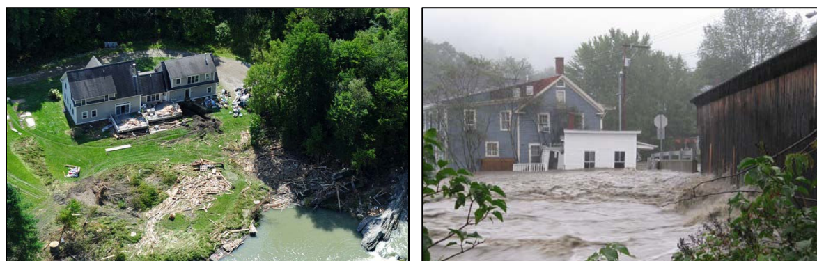
Figure 2. These images show the flood damage in the Mad River Valley from Tropical Storm Irene: a damaged home along Vermont Route 100 adjacent to Moretown Village (left) and a damaged building in Waitsfield (right). Credits: Lars Gange and Mansfield Heliflight (left), Jeff Knight, The Valley Reporter (right).
