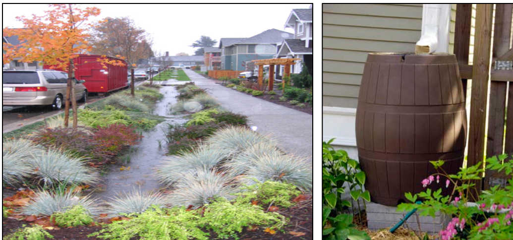
Figure 15. Green infrastructure techniques such as rain gardens (left) and rain barrels (right) retain stormwater runoff on site and reduce peak flooding. Credit: Clarion Associates.
