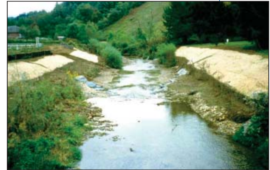
Figure 11.6 Cove Creek after restoration
