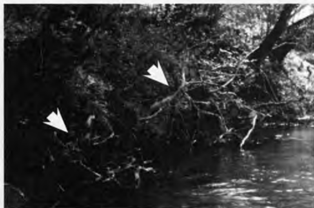
Figure 2. Root wads after installation.
