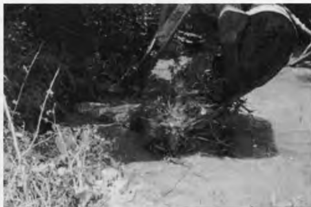
Figure 3. Root wad installation using drive-point method.
