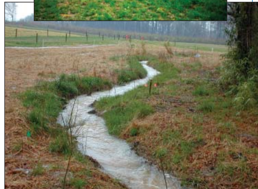
Figure 5.7 Yates Mill Pond tributary-restoration project after construction
