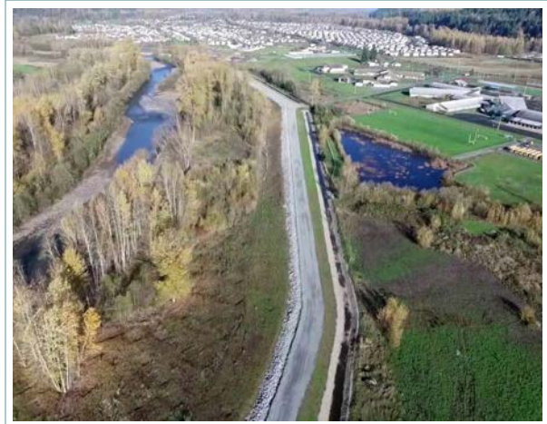
Calistoga Reach floodplain restoration in Washington. Photo: CSI Drone Solutions and Washington Rock Quarries, Inc.
