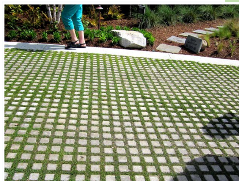
Permeable paver patio can increase infiltration and reduce stormwater runoff. Photo: ECV-OnTheRoad
