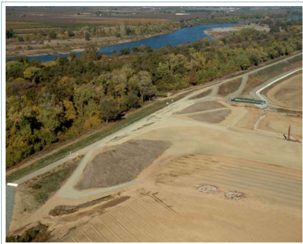
Bear River setback levee in California. Photo: California Department of Water Resources
