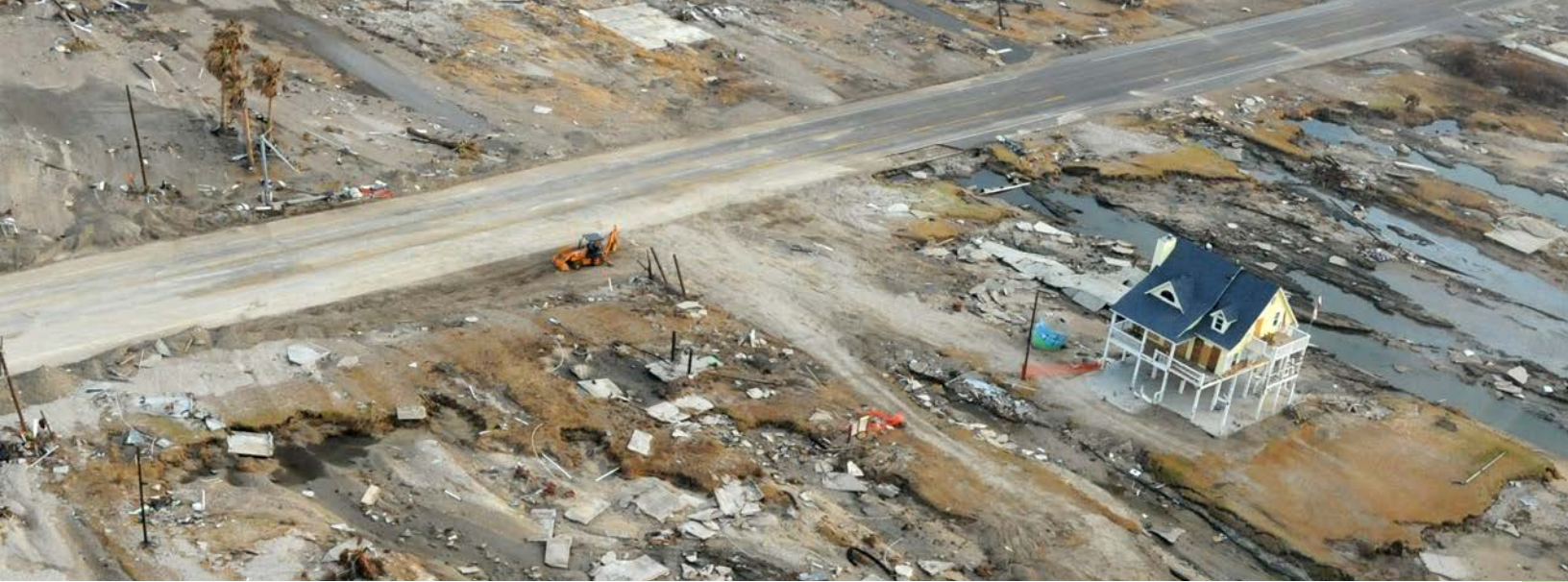
Damage from Hurricane Ike in Texas in 2008. Photo: Federal Emergency Management Agency
