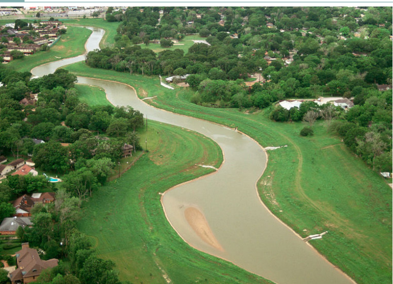
Restoration of Sims Bayou in Houston, Texas consisted of earthen channels and tree plantings to reduce flood risks. Photo: SWA Group
