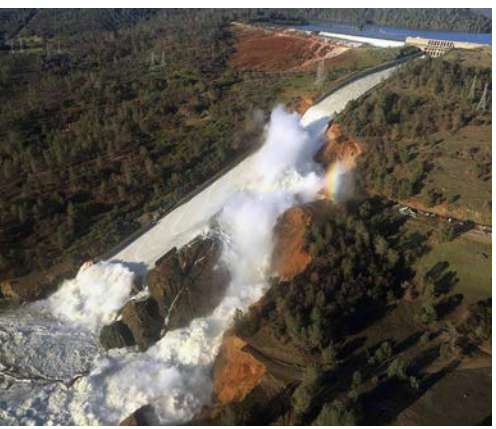
2017 Oroville Dam spillway failure in California. Photo: William Croyle/California Department of Water Resources
