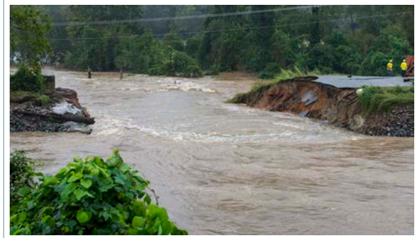
Levee breach in Columbia, South Carolina. Photo: U.S. Air National Guard
